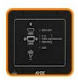
The staff inputs are on panels that are located on the left and right walls above the half-wall separating the gallery from the well of the courtroom. The Large Courtrooms have a third staff support input panel that is in the center of the half-wall. You may select either the VGA or HDMI input from these locations.
